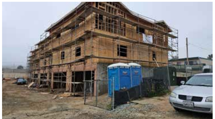
Off of Santa Fe, glimmer of hope. This complex has garages!
