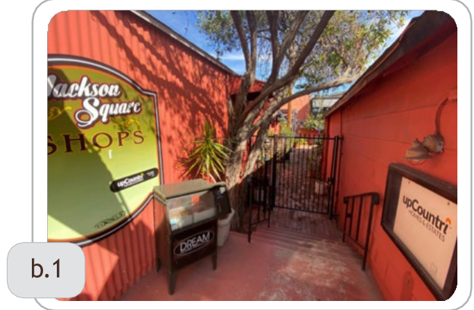
Alley between buildings showing consistent façade
