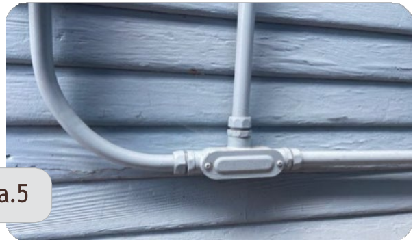
Surface mounted utility conduit
