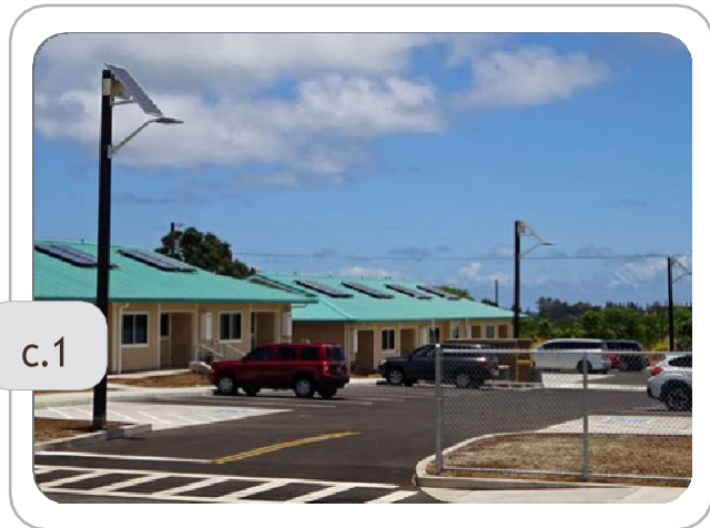
Example of overhead fixtures for pedestrian areas
