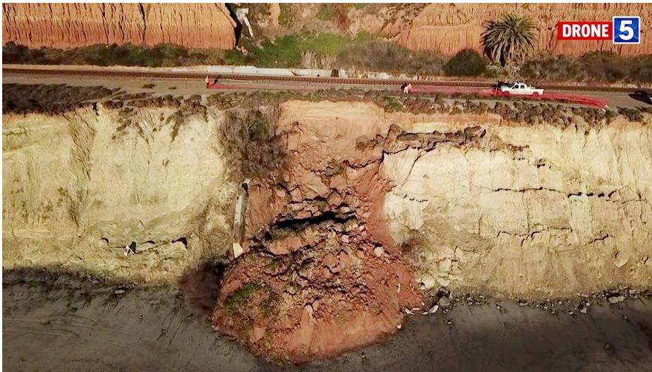
BLUFF COLLAPSE SANDAG REPAIR PILINGS FAILURE
